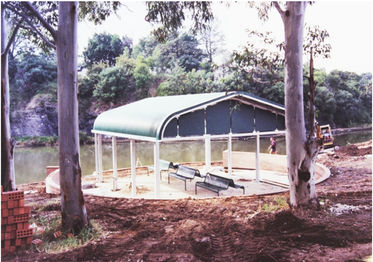
Queens Wharf Construction, 1988.
