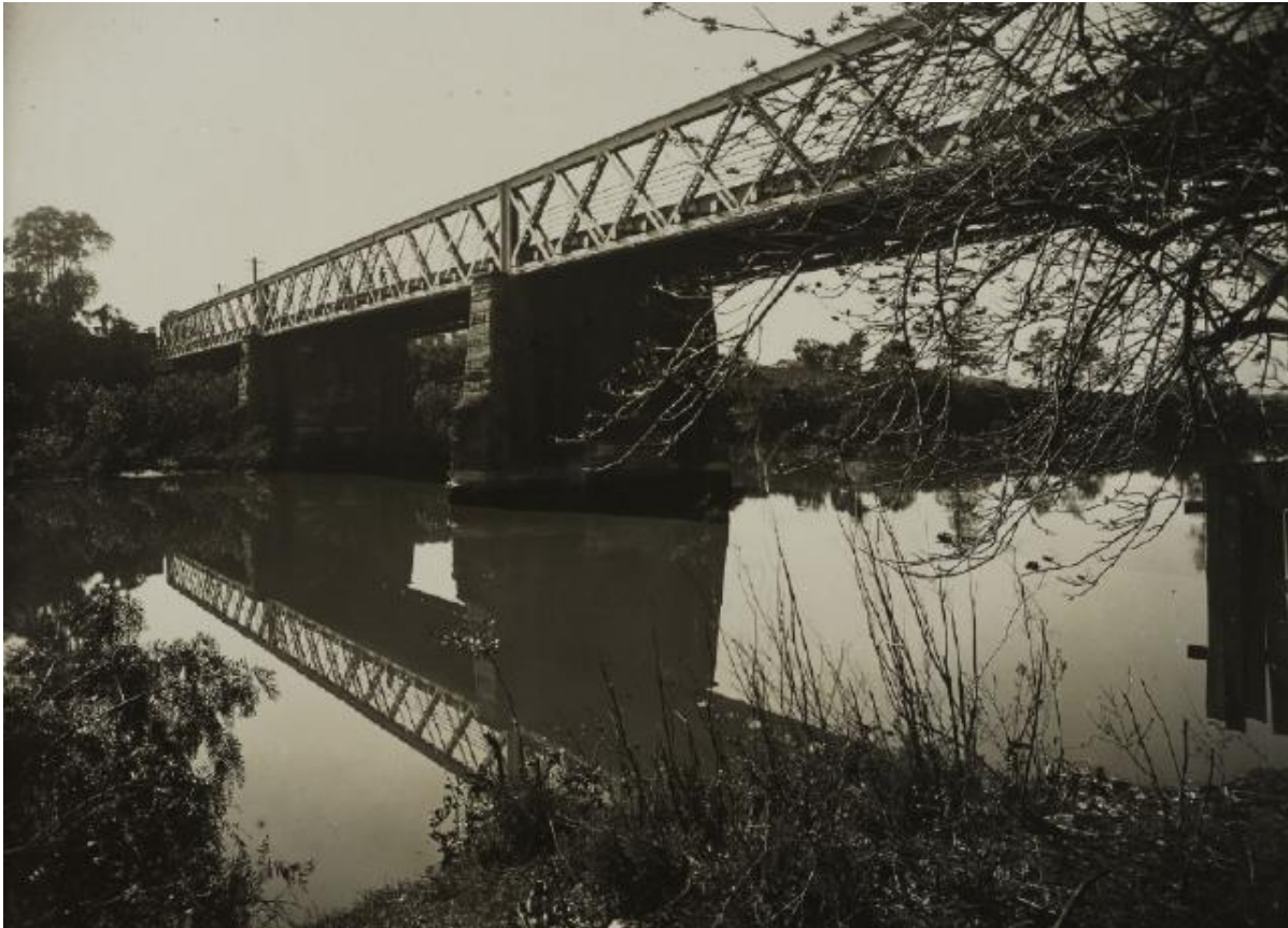
Gasworks Bridge, Parramatta, view of bridge from a low position on an adjacent river bank, circa 1928.
