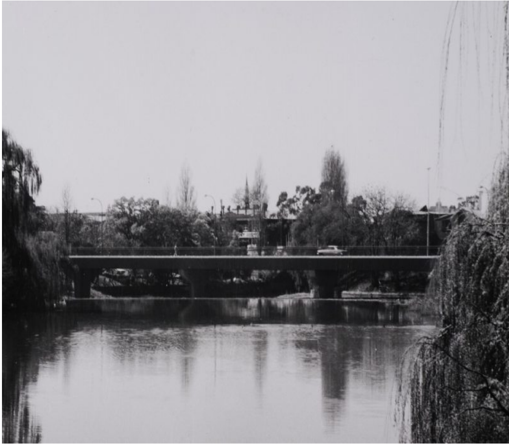
Marsden Street Bridge, Parramatta, 1972, (now Bernie Banton Bridge).
