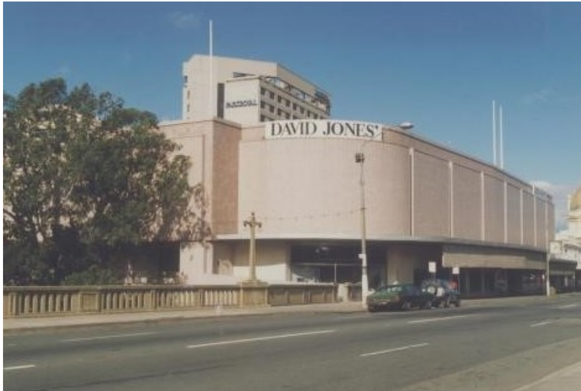
David Jones Building, 1992.
