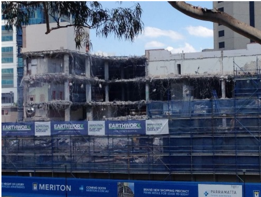
Demolition of David Jones building November 2013.
