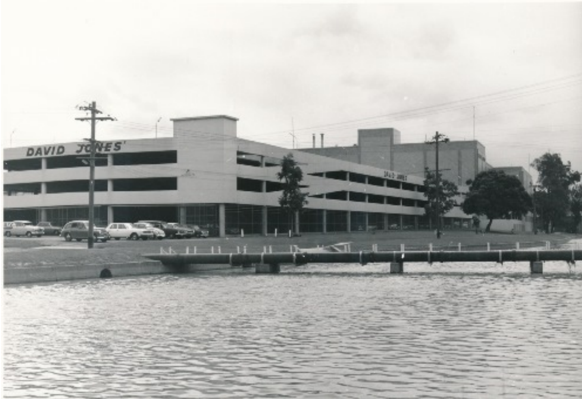
David Frater Reserve Car Park. Airspace leased to David Jones. View to the south west 1969. Source: City of Parramatta Council Archives
