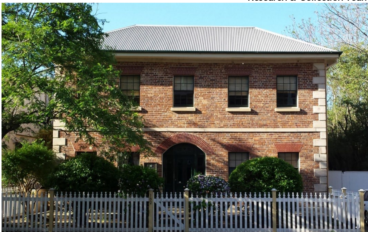
Harrisford House, George Street, Parramatta, 2014. Source: Geoff Barker, Parramatta City Council
