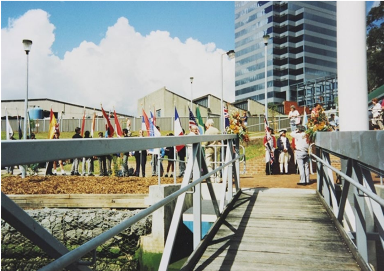
Queens Wharf Construction, 1988.
