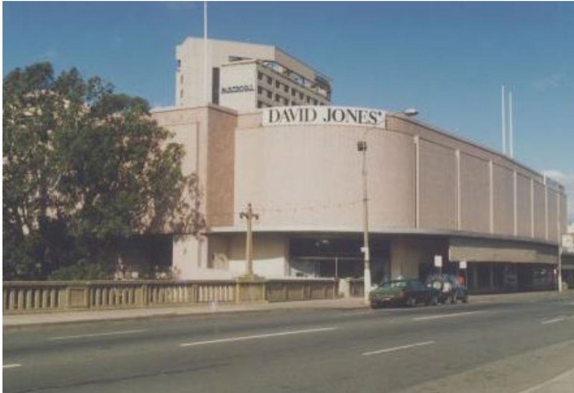
David Jones Building, 1992.
