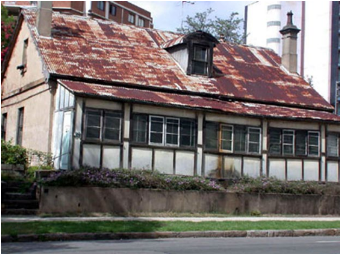
Lennox House 39 Campbell Street, Parramatta.
