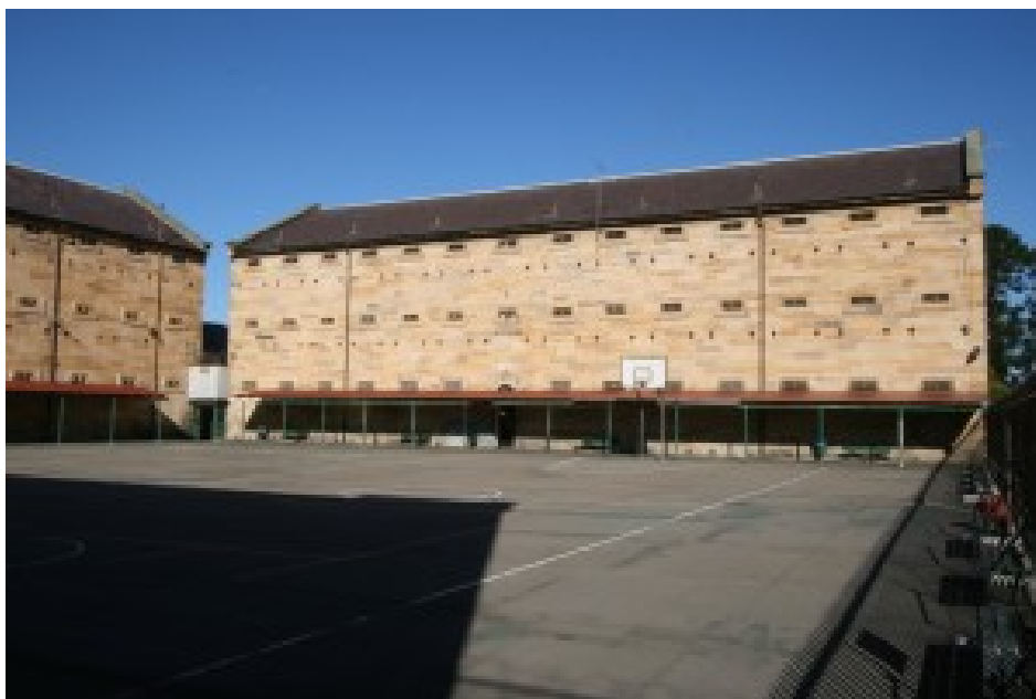
Parramatta Gaol Sports Yard, 2012. (Source: Geoff King, Parramatta City Council).
