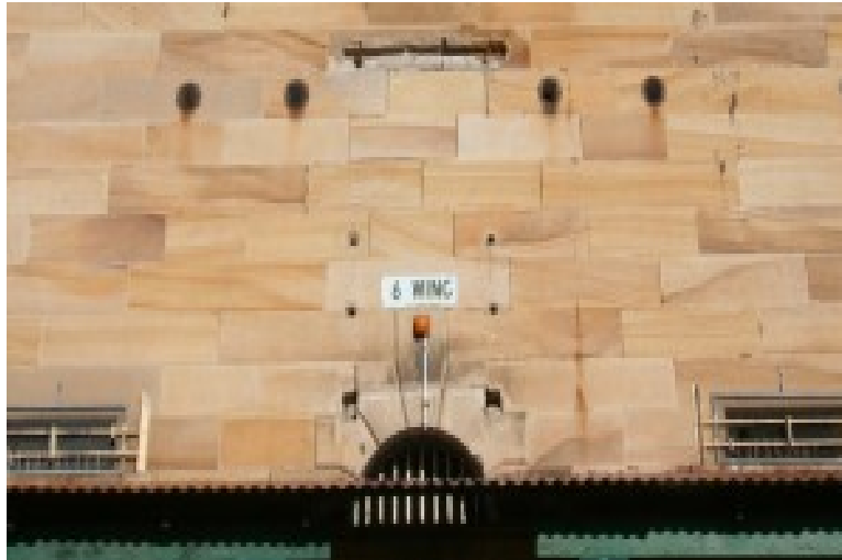
Parramatta Gaol Six Wing, 2012. (Source: Geoff King, Parramatta City Council).
