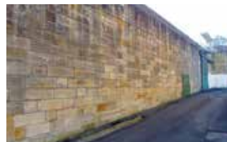
P 25a Sandstone Perimeter and Compound Walls constructed over a number of stages (1837, 1863 and 1880s)
