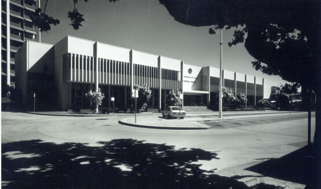
Parramatta City Library 1979 following its expansion. Parramatta Council Archives
