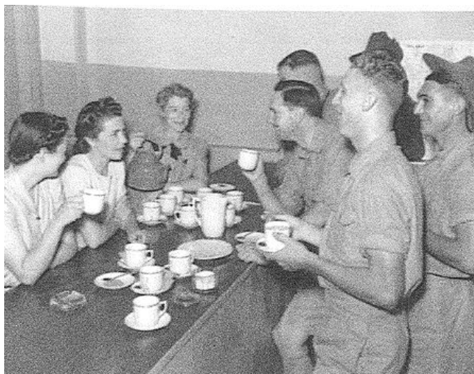
The interior of an Australian WW2 soldiers' hut, similar to the one that opened in Parramatta in 1940. Image: Australian War Memorial, Acc no. 002120
