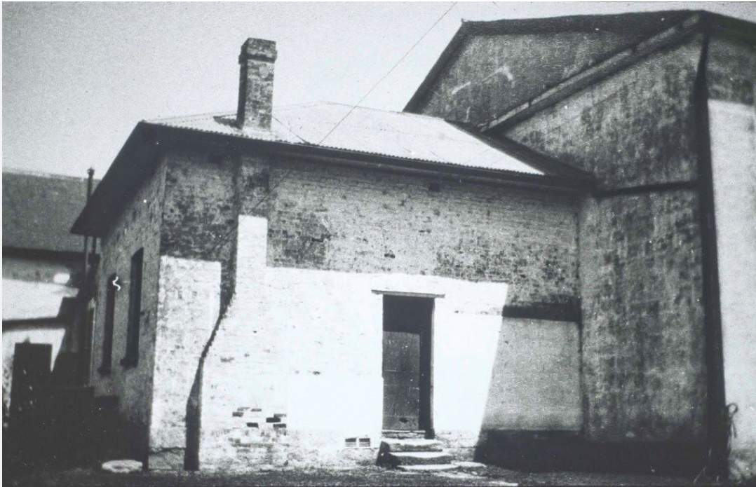
Old Lawry Chapel building, rear of Macquarie Hall, Macquarie Street, Parramatta City Council, Heritage Centre, LSP00185
