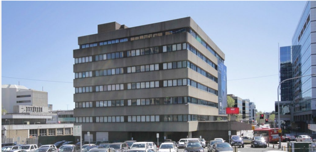
Rear of Macquarie House Corner of Macquarie and Smith Streets. Source: Macquarie House Archival Recording 2014
