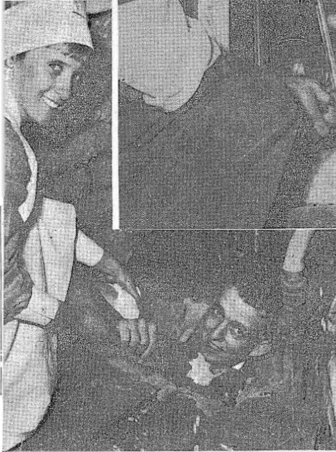
ABOVE: An Argus reporter examines by the light of a hurricane lamp; the rotting timbers beneath the floor of the nurses' home in Parramatta. Picture at left shows the reporter being helped from the cellar by Nurse Sandra Shaw. During wet weather the cellar is flooded, sometimes to a depth of 14 inches.
