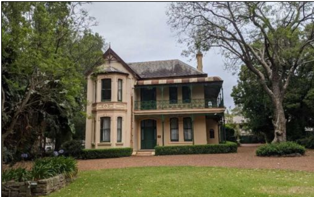
Figure 2-1 Looking north-east to Willow Grove from the front garden (Source: Advisian, 2020).
