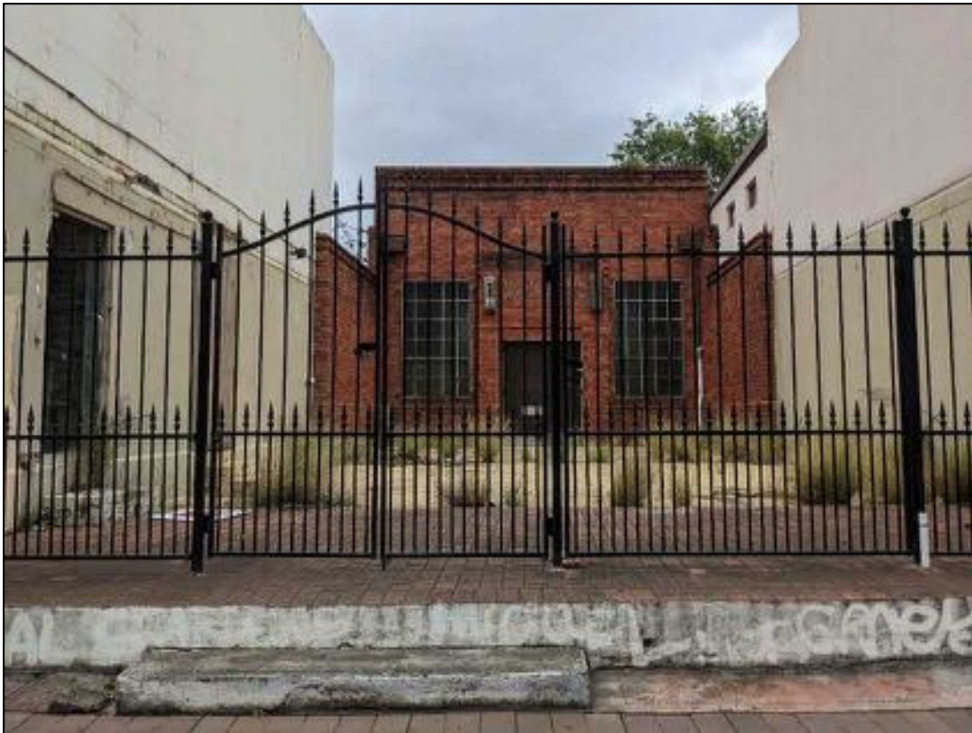
Figure 4-1 Looking north-east to P & G E S Co. Ltd. Sub-Station No. 16 from Phillip Street (Source: Advisian, 2020).
