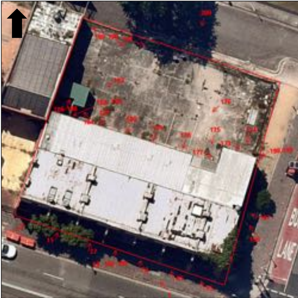
Figure 3-4 Locations and angles of external photographs taken at St George's Terrace (Source: Nearmap, 2020, as modified by Advisian).
