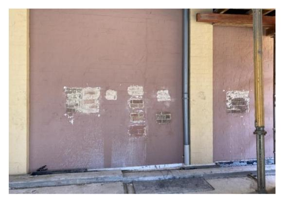
Northern elevation of the Town Hall during paint stripping tests. Note the bricked up arched openings.
