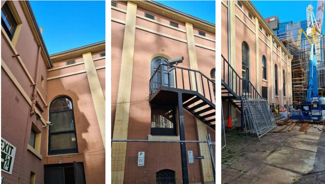
52 South elevation of the Town Hall showing numerous modifications made to windows and doors. The 1932 addition is shown in the photo to the far left. Source: TKD Architects.
