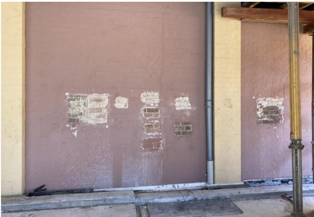
50 Northern elevation of the Town Hall during paint stripping tests. Note the bricked up arched openings.
