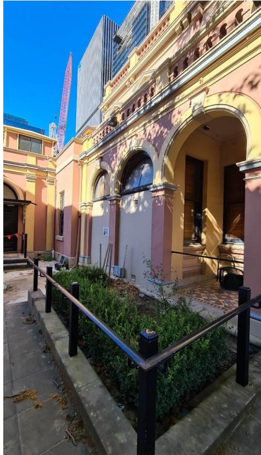
47 Jubilee Hall western elevation and main entry doors (left) and northern elevation of the former Council Chambers (right). Note the enclosed arches to G02. A concrete ramp leads from the front verandah to the Jubilee Hall entrance.
